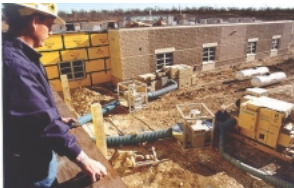
Figure 4. Drying during construction.
