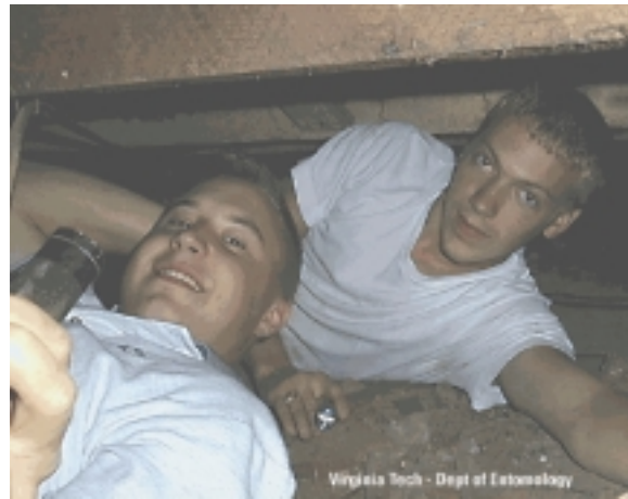
Figure 11. Investigations of crawl spaces would be easier with a portable mold detector which could locate mold from the occupied side of the 1st floor rather than from below.
