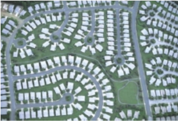
Figure 6. When houses are close together, rainwater from roofs can collect between them, leading to drainage problems and water near the foundations.
